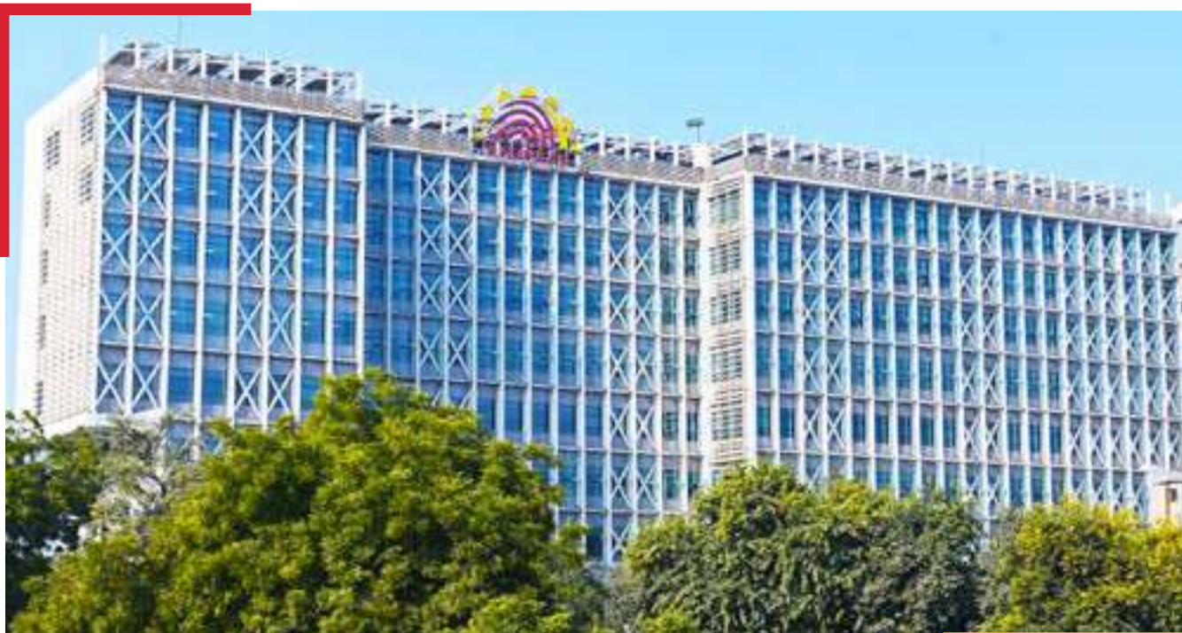
UIDAI HQ Building, New Delhi
